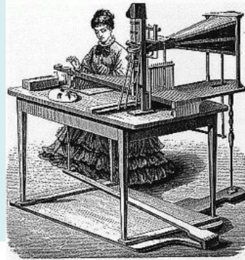
A drawing of The Euphonia, an early mechanical speech synthesis machine
